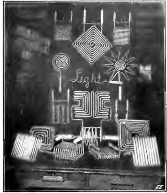
Fig. 4. This photograph represents a collection of a few of Tesla's wireless lamps, such as he proposes to use in lighting isolated dwellings all over the world from central wireless plants. The two lamps at either corner at the bottom are illuminated, owing to the fact that a high frequency oscillator was in operation some distance away when this photograph was being taken. These tubes were filled with various gases for experimental research work in determining which was most efficient.
